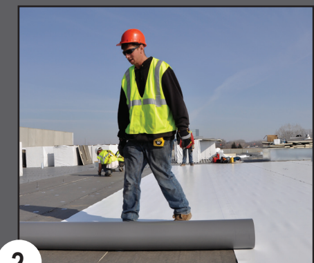
2 Apply membrane, overlapping seams in the direction of water run-off.
