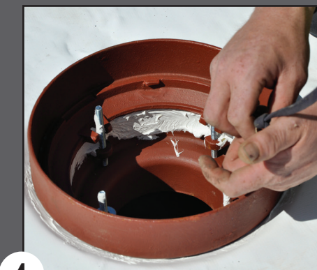
4 Seal free edges of membrane with urethane sealant.
